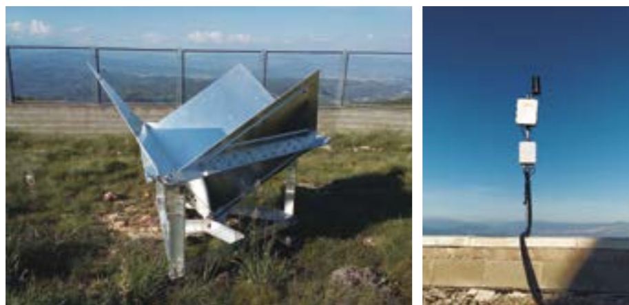
Figure 2: Corner reflector for the calibration of the Sentinel-6 satellite installed at the OdM (left); i2Cat antenna for IoT communication testing installed at the OdM (right).
