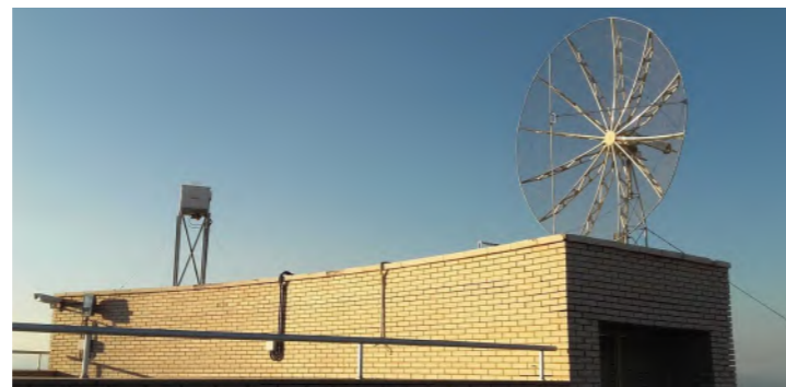
Figure 13: S-Band antenna installed at Montsec Astronomical Observatory facilities.
