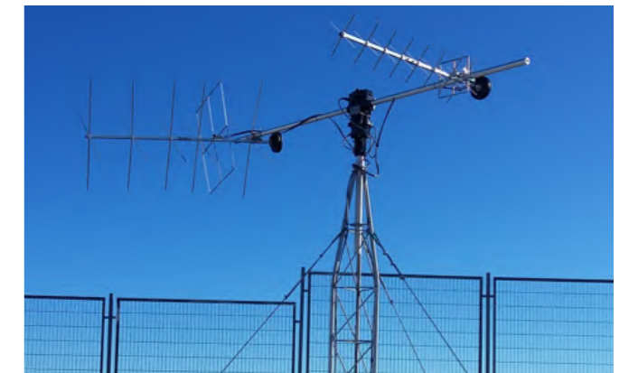
Figure 8: VHF/UHF ground station antenna.
