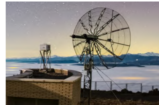
Figure 7: S-band ground station antenna (with the AllSky Camera visible to its left).
